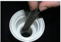
If hole is blocked with glue or pipe shavings use a file or knife to trim until the Pool Valet Retro nozzle will fit into the pipe.
